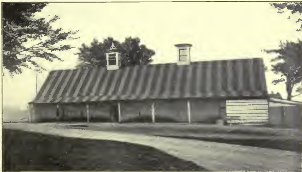
OLD GUARD-HOUSE IN AMERICAN REVOLUTION—Photograph taken at the ancient structure known as the Carlisle Barracks and built in Pennsylvania by Hessians captured at the Battle of Trenton in New Jersey.
